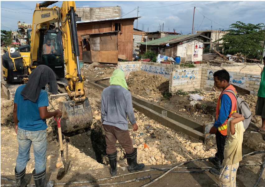
Building New Homes in Paknaan, Mandauae
